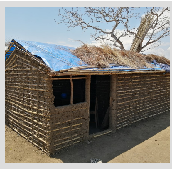
Figure 2: Construction of Permanent Houses in Tratara Sites
