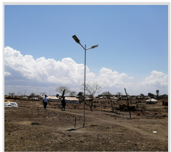
Figure 6: Lighting in a common space-Tratara site
