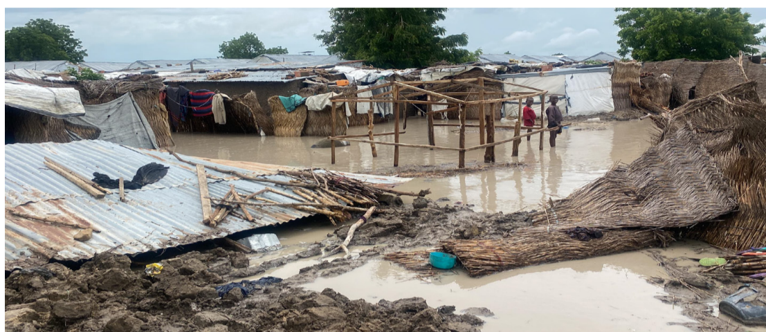
Picture showing damaged shelters after the heavy rainfall © IOM 2024
