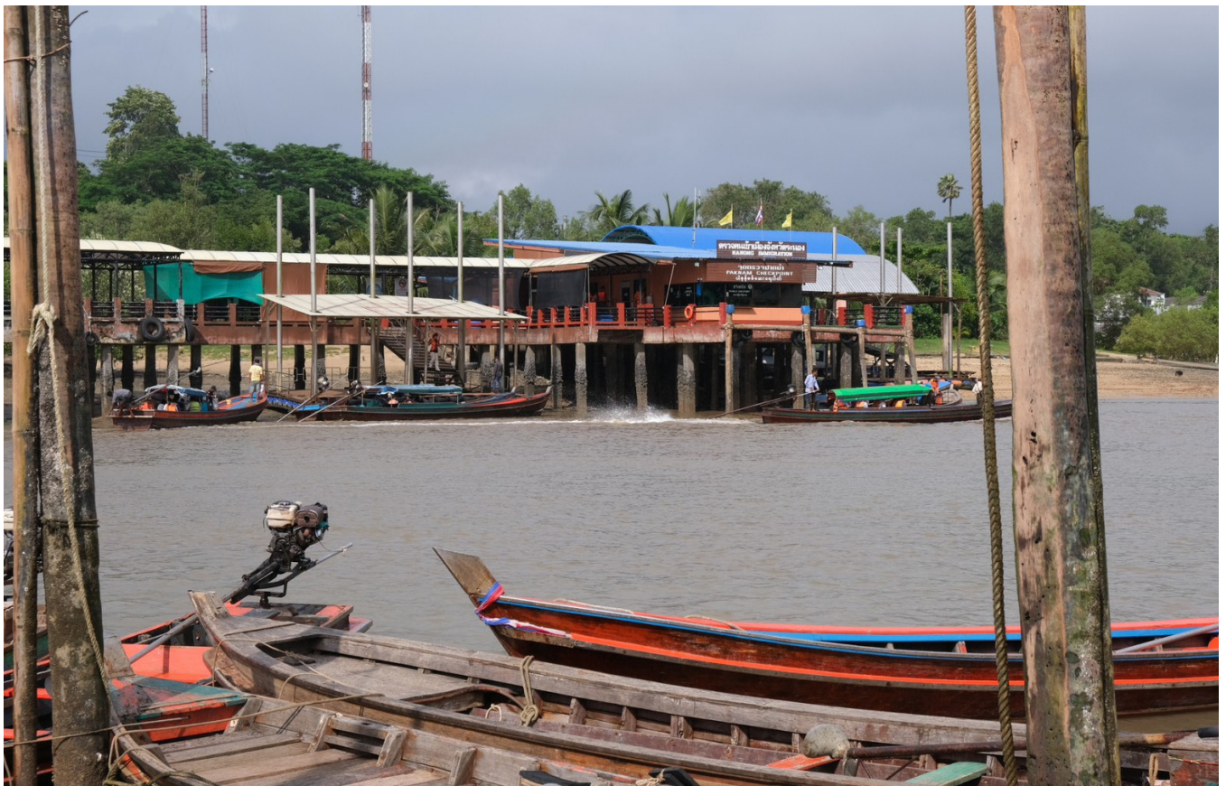
PHOTO Pak Nam checkpoint, where people must stop to register before entering Ranong through Saphan Pla POE. © IOM 2023/Somruedee KARNPHAKDEE
