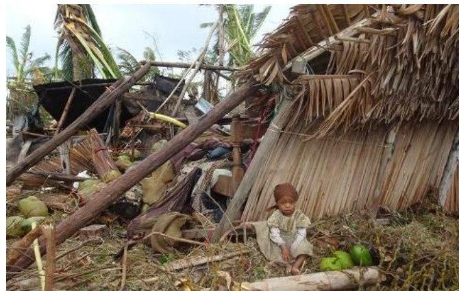
Figure 4 Damaged housing, 8 March 2017 (CARE Madagascar)
