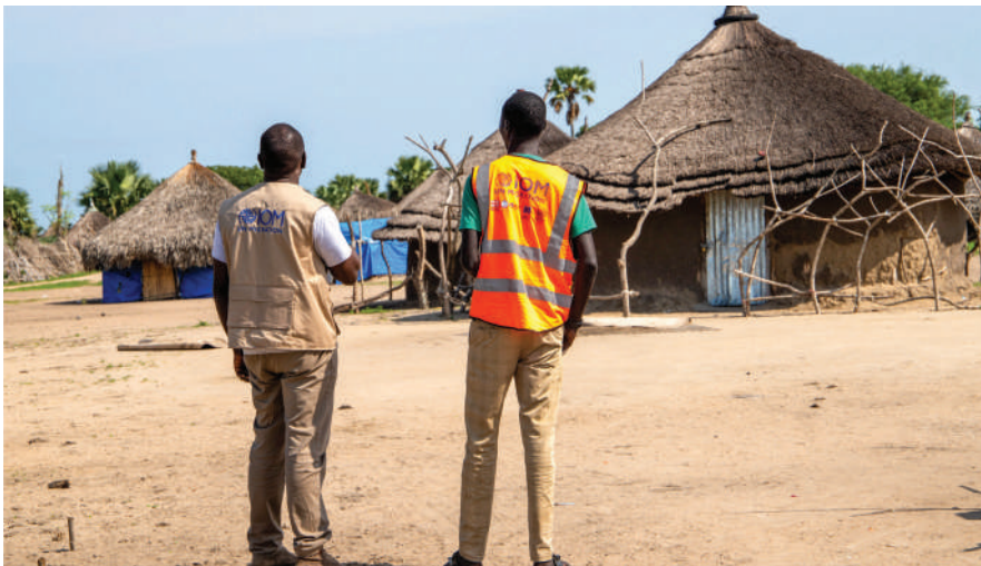
The most common shelter type is mud wall with grass thatched roof.
