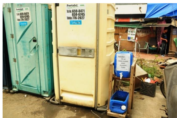
Portalets at Streetlight EC at Tacloban City
