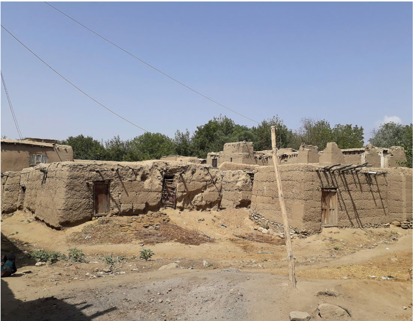
Despite having access to electricity, families in Nejrab district are suffering from poor living conditions. The shelter shown in this picture is not only old but also unreliable. © IOM 2018
