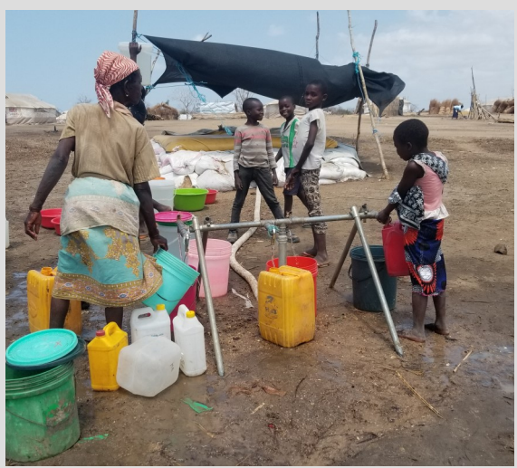
Figure 3: Small water system in Tratara RS-Water Truck
