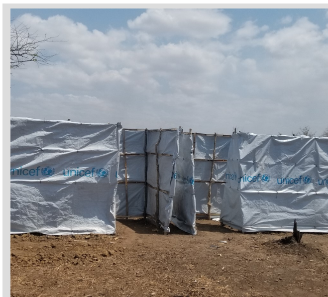
Figure 4: Latrines in Chuiba Transit Centre
