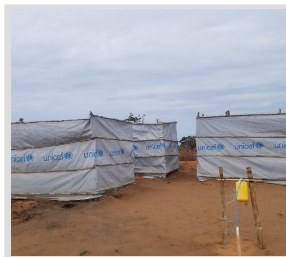
Figure 4: Handwashing station near latrines - Chuiba
