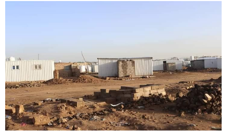
Different construction techniques at Al Jufaina IDP camp affected differently from heavy rains. DTM Marib. Dr Hassan Al Hassani.
