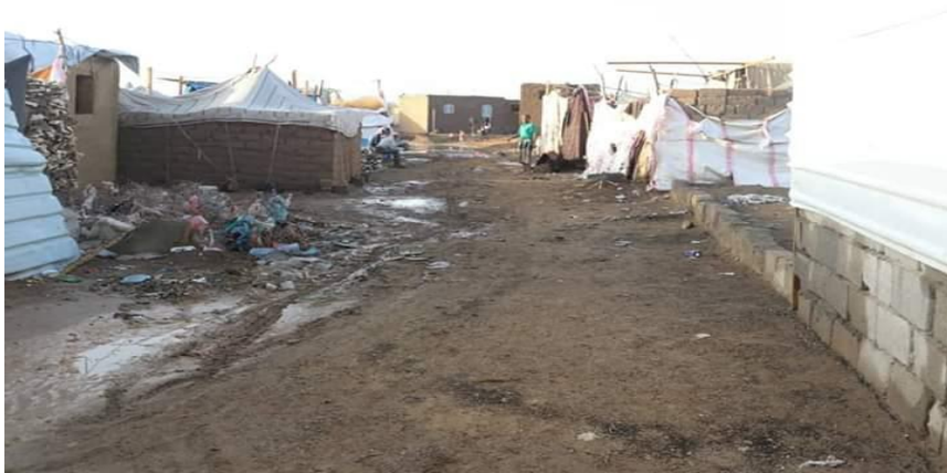
House wall in Al Jufaina IDP Camp destroyed from heavy rain. DTM Marib. Dr Hassan Al Hassani.
