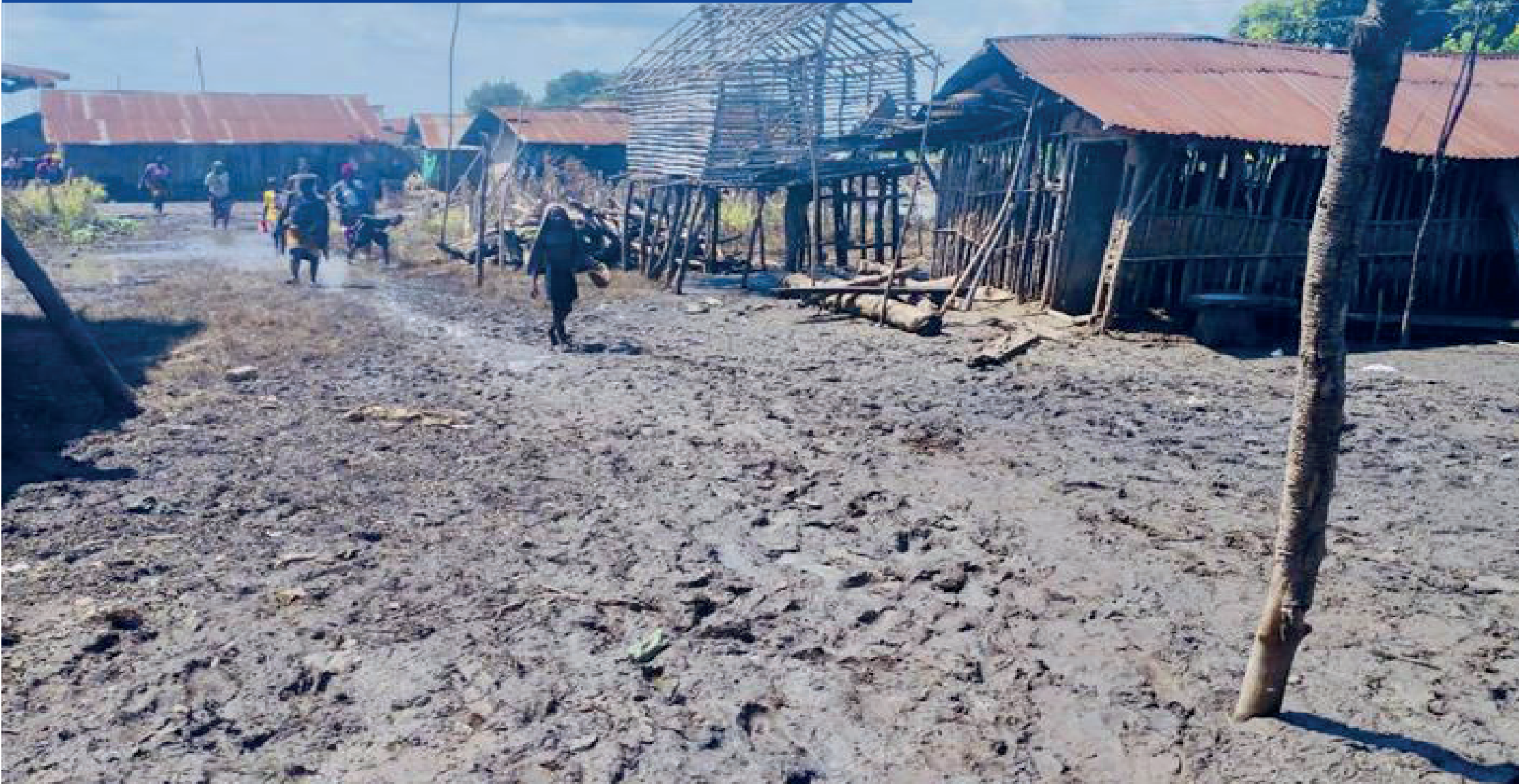
A shelter in ruins after the flooding in Esan South East LGA of Edo State © IOM Nigeria / Kingsley IYERE
