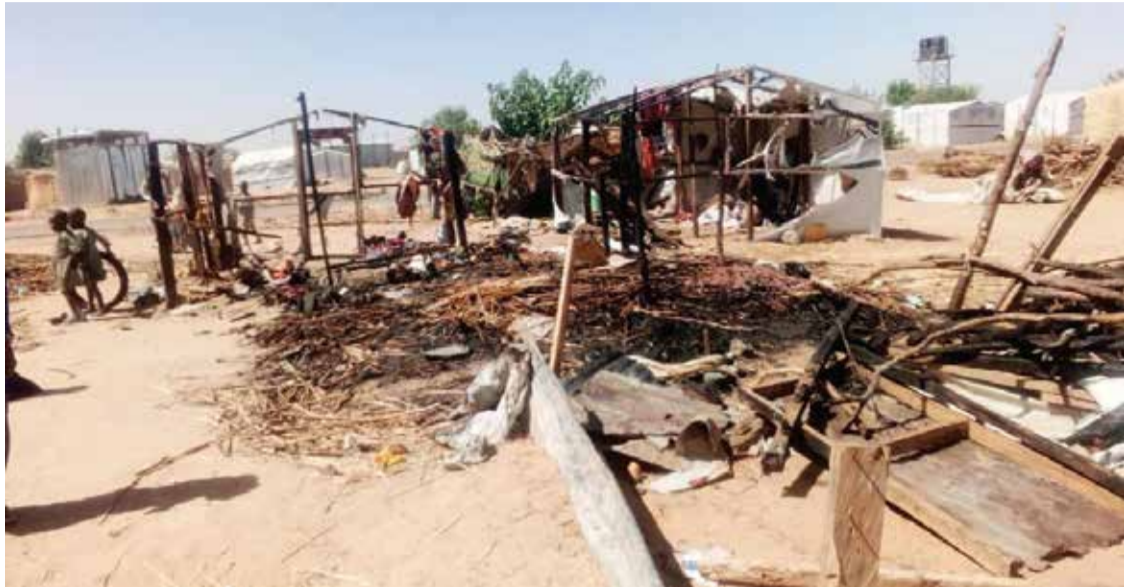
Picture showing damaged shelters after the fire outbreak © IOM 2024
