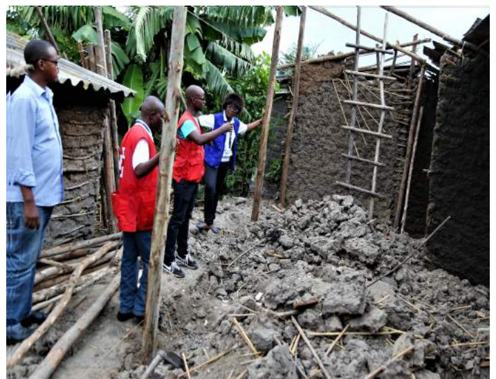
Photo 5: IDP home partially destroyed by torrential rains. Bubanza province, Gihanga commune © IOM 2018.
