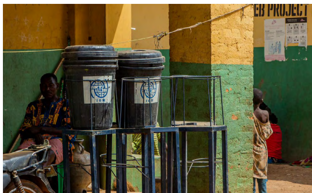
A newly installed hand washing station for IDPs in Ortese camp, Guma LGA of Benue State © IOM Nigeria / Phoebe Awosina / IOM 2022
