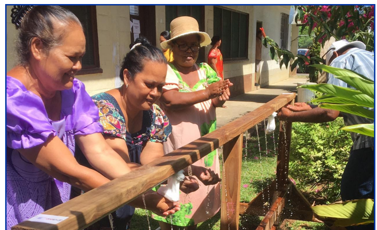
Hand washing station installed in Chuuk, FSM.
